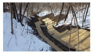
Installation of erosion control blanket in completed section of stream
