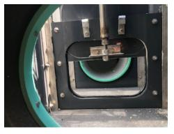
Photograph of inside the water level control structure. Photograph is taken looking upstream towards where water comes into the filter. The structure consists of a solar panel (not shown), control panel (also not shown), and the gate. The control panel is programmed to open and close the gate on a schedule that staff program.
