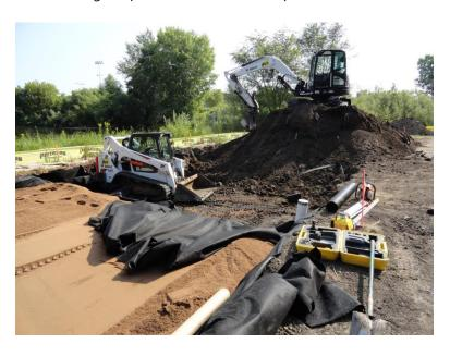
Iron-enhanced sand filter excavation.
