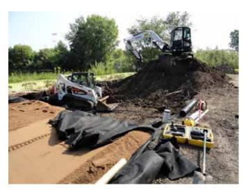
Photo of the iron enhanced sand filter installation
