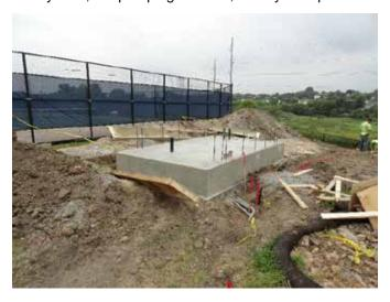
Photo of the water treatment shelter foundation, after forms removed
