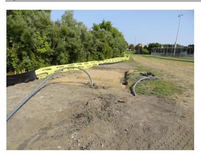
Pump pad foundation (has since been re-excavated to remove additional subgrade soils) and directionally drilled HDPE.
