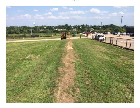
Low voltage communication line in Magellan Easement from treatment shelter to existing irrigation box/controls
