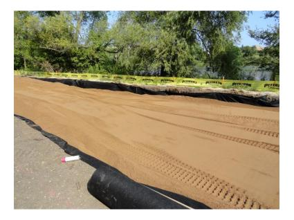
Iron-enhanced sand filter post excavation, geotextile placement and iron-enhanced sand backfill.
