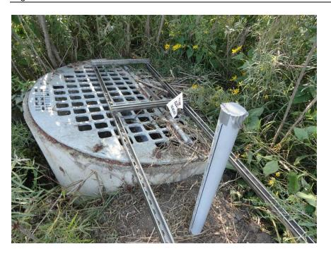
Line for water level sensor at existing pond outlet structure
