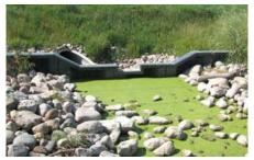
Example of a stage weir from the *Minnesota Wetland Restoration Guide* by the Minnesota Board of Water and Soil Resources (BWSR)
