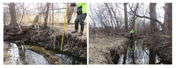
Figure 4-1 Incised and straightened channel in Sub-Reach B5B
