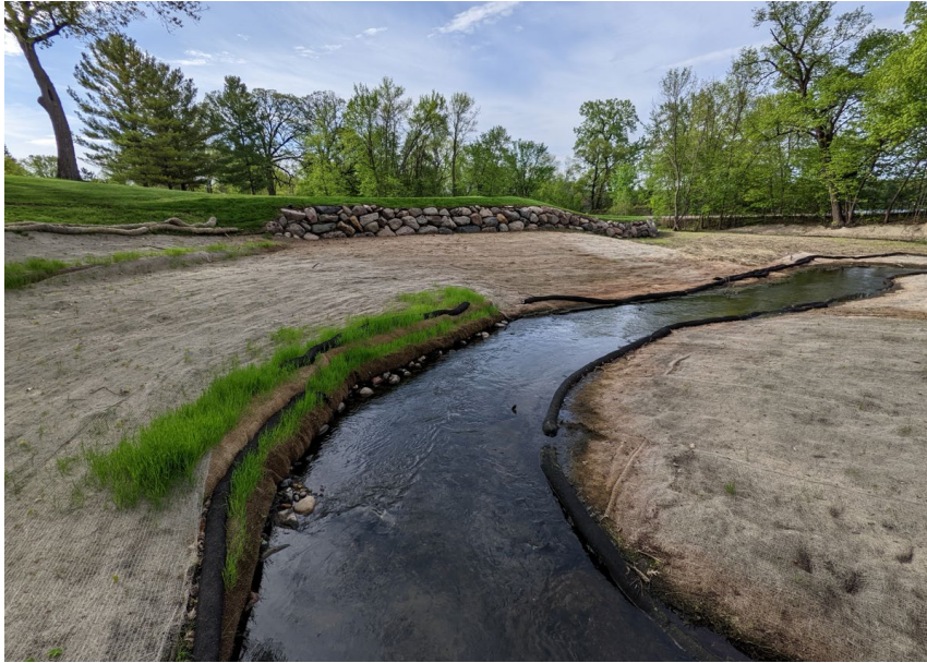
Photo of south site, looking downstream at VRSS on left bank and realigned channel
