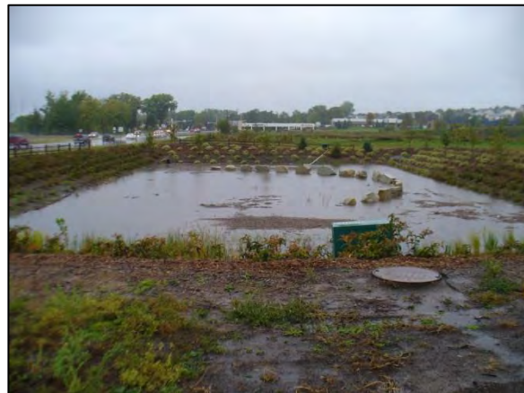
Iron-enhanced sand filtration system near Beam Avenue following a rainfall event (Ramsey-Washington Metro Watershed District, 2017).
