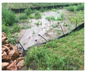
District staff inspect project sites and direct permit holders to take corrective actions as needed to protect water quality. The image above shows a silt fence violation (failure) at a site in 2021.
