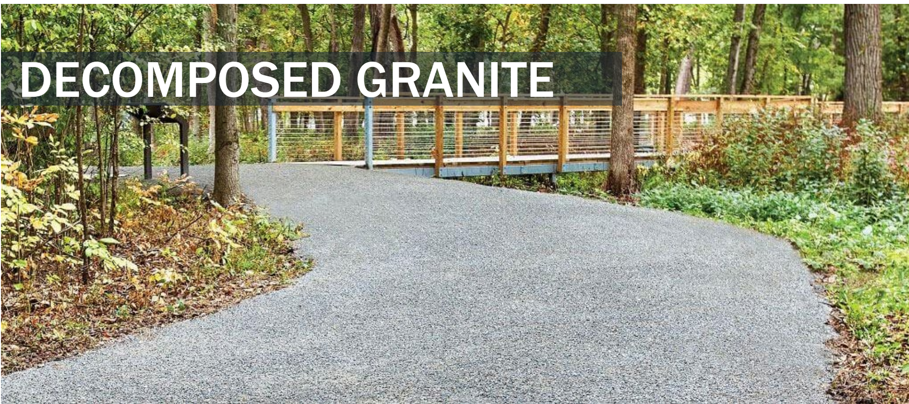
DECOMPOSED GRANITE Trail Surfacing A combination of granite aggregate and fines bound with a natural stabilizer to create an ADA accessible surface
