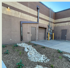
AFTER: A downspout is redirected to a rain garden
